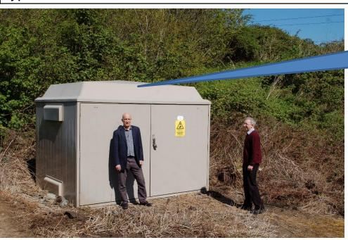
Flat profile antenna mounted on roof of GRP cabinet
